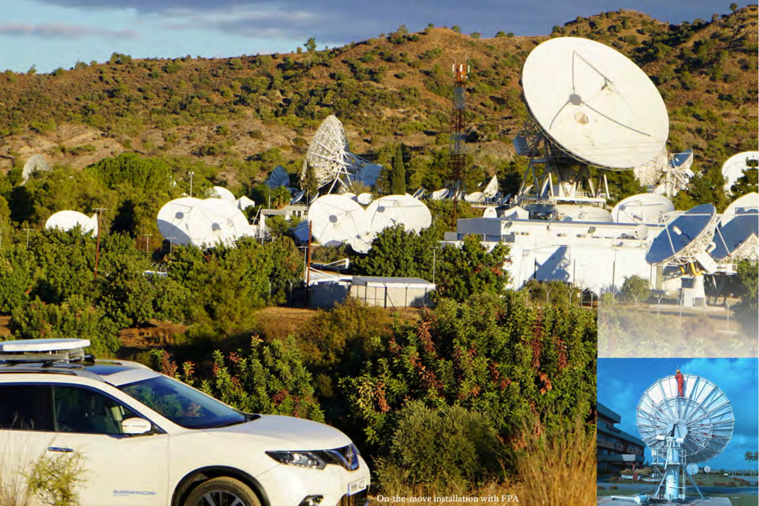
On-the-move installation with FPA
