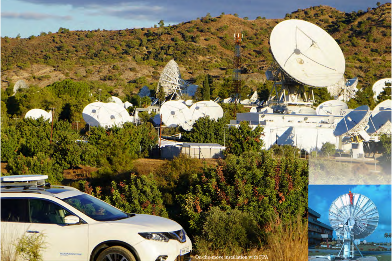
On-the-move installation with FPA
