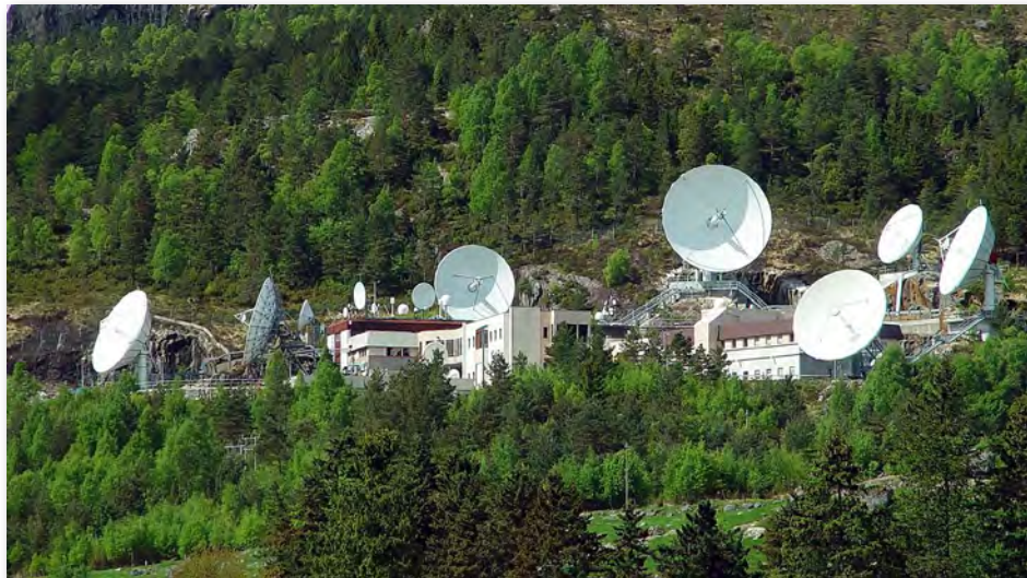
Marlink's Eik receiving station.
