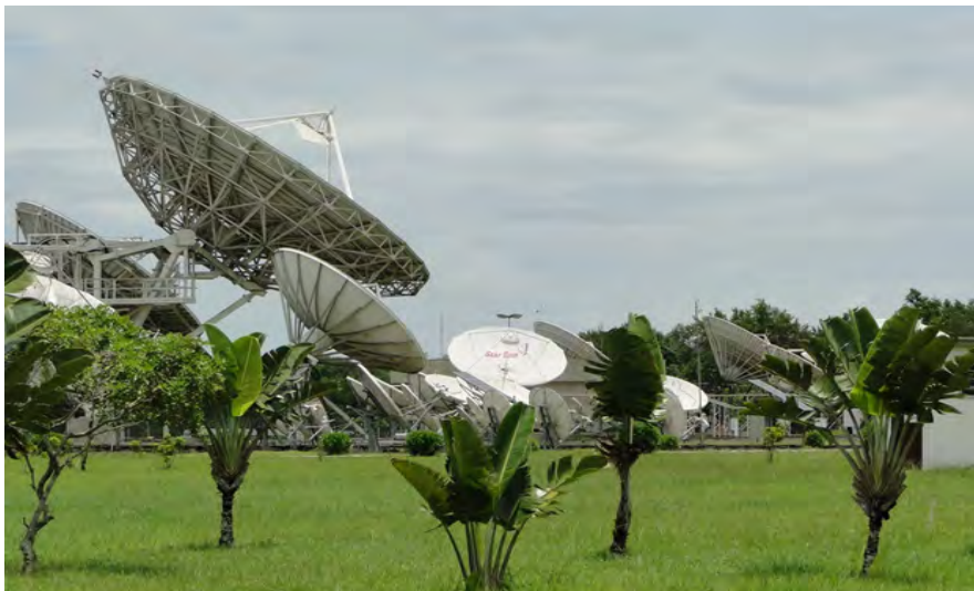
Hispamar's Guaratiba Satellite Control Center in Rio de Janeiro, Brazil
