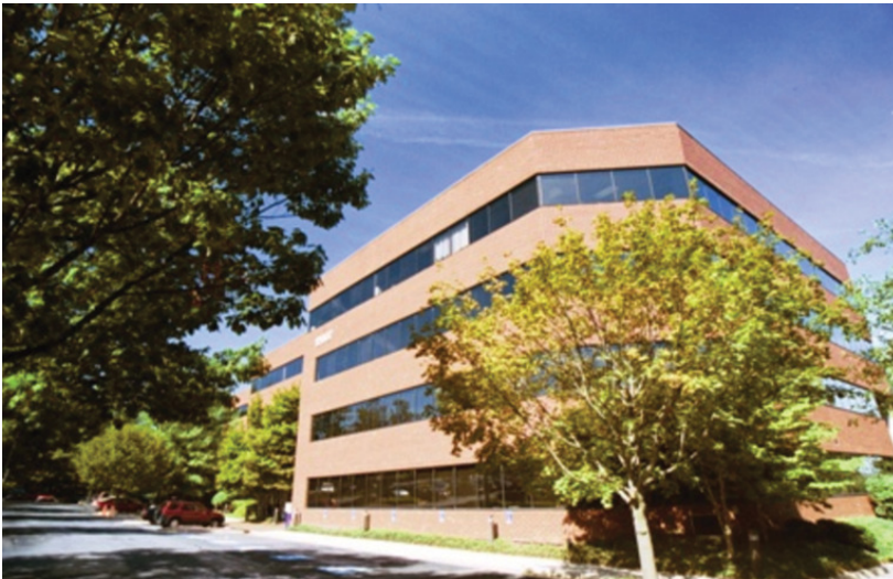
Revgo Global's headquarters and main R&D facility in Reston, Virginia, USA. Revgo Global also has facilities in Houston, Texas and in Guangzhou, China.
